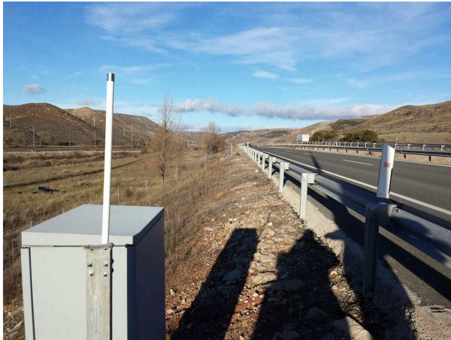
Figure 6: Roadside ITS-S in the A-2 highway
