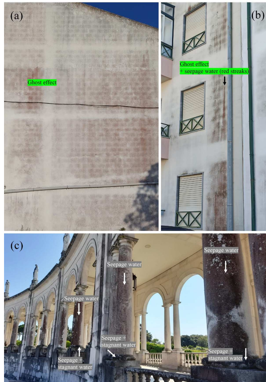
Figure 4. Practical case of bio-colonization as markers of building pathologies: (a,b) private buildings, (c) colonnade at Fatima's sanctuary.
