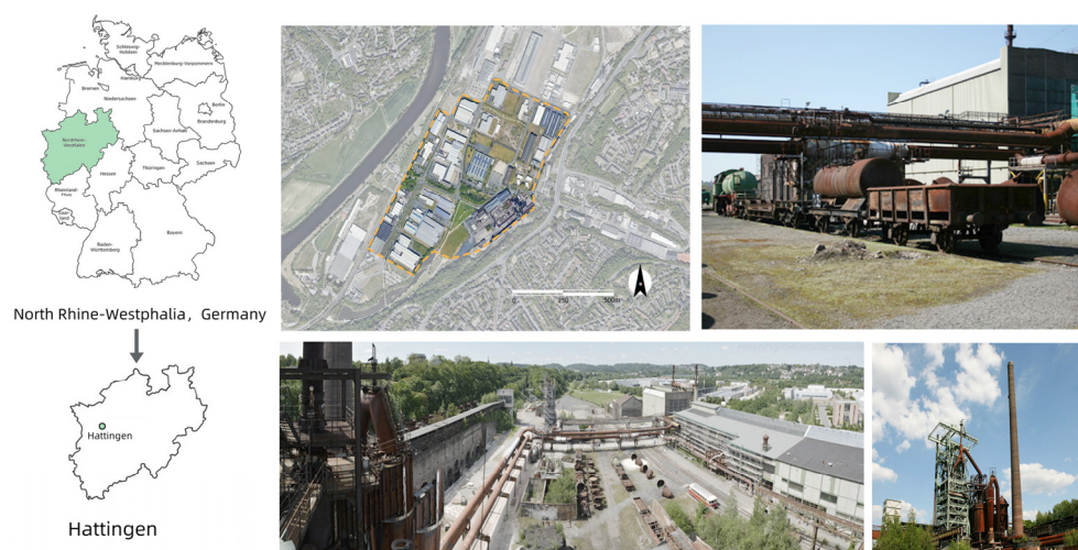
Figure 8. Location and current status of Henrichshutte.
