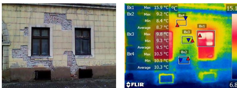
Figure 26. Thermogram of the probing building part of a known wall structure.
