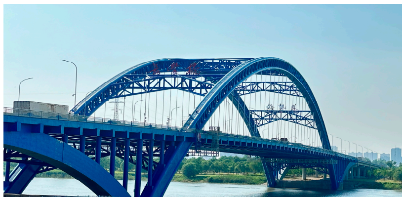
Figure 2. Overview of the bridge.
