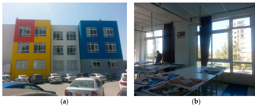
Figure 6. (a) Northeast façade; and (b) internal view from the northeast facade.
