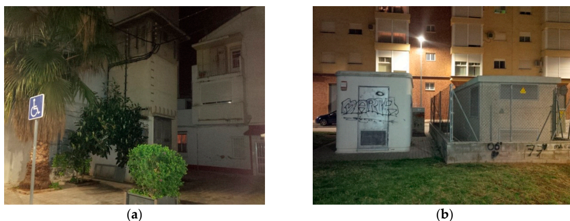
Figure 1. The oldest and most recent TS where it has been measured: (a) Tower with very old TS, more than 60 years old; (b) Precast concrete box with very recent TS, less than 10 years old.
