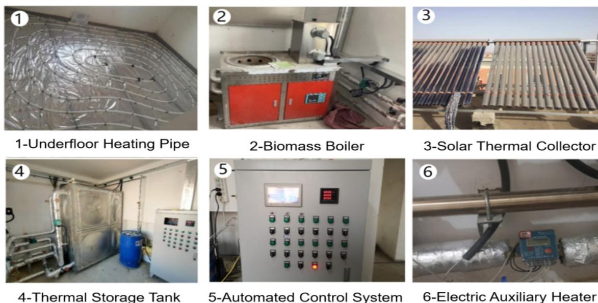
**Figure 2.** The MECH System equipment diagram.
