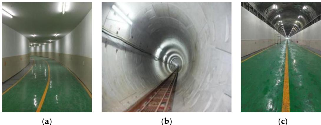
**Figure 2.** Types of corridors in actual engineering. (a) Rectangular tunnel. (b) Circular tunnel. (c) Arch tunnel.
