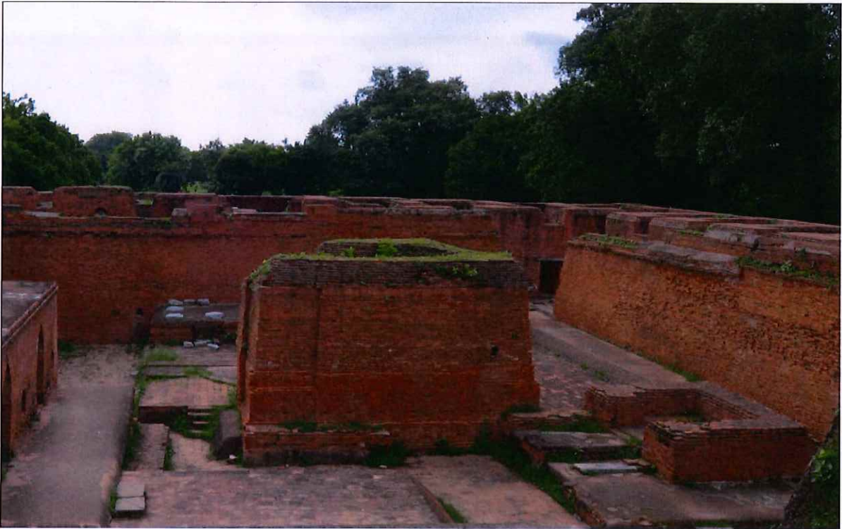
Structural Conservation at Monastery 1 (before)
