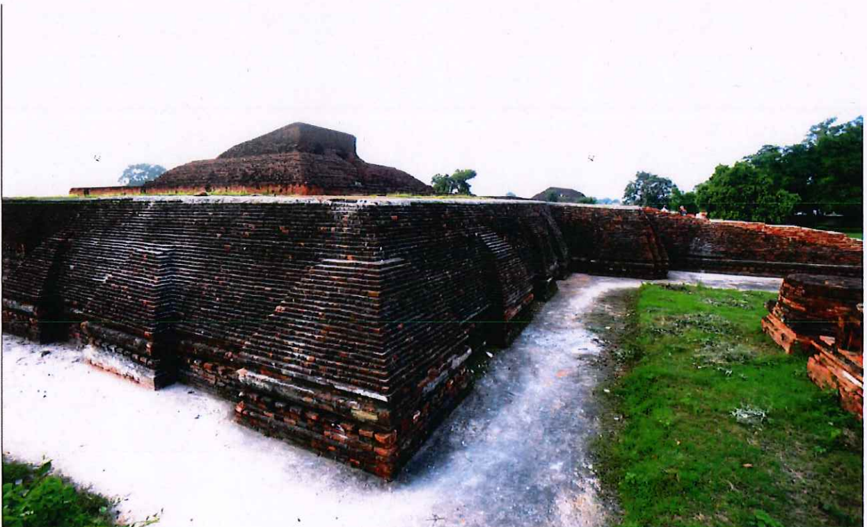
Structural Conservation at Temple site 13 (after)
