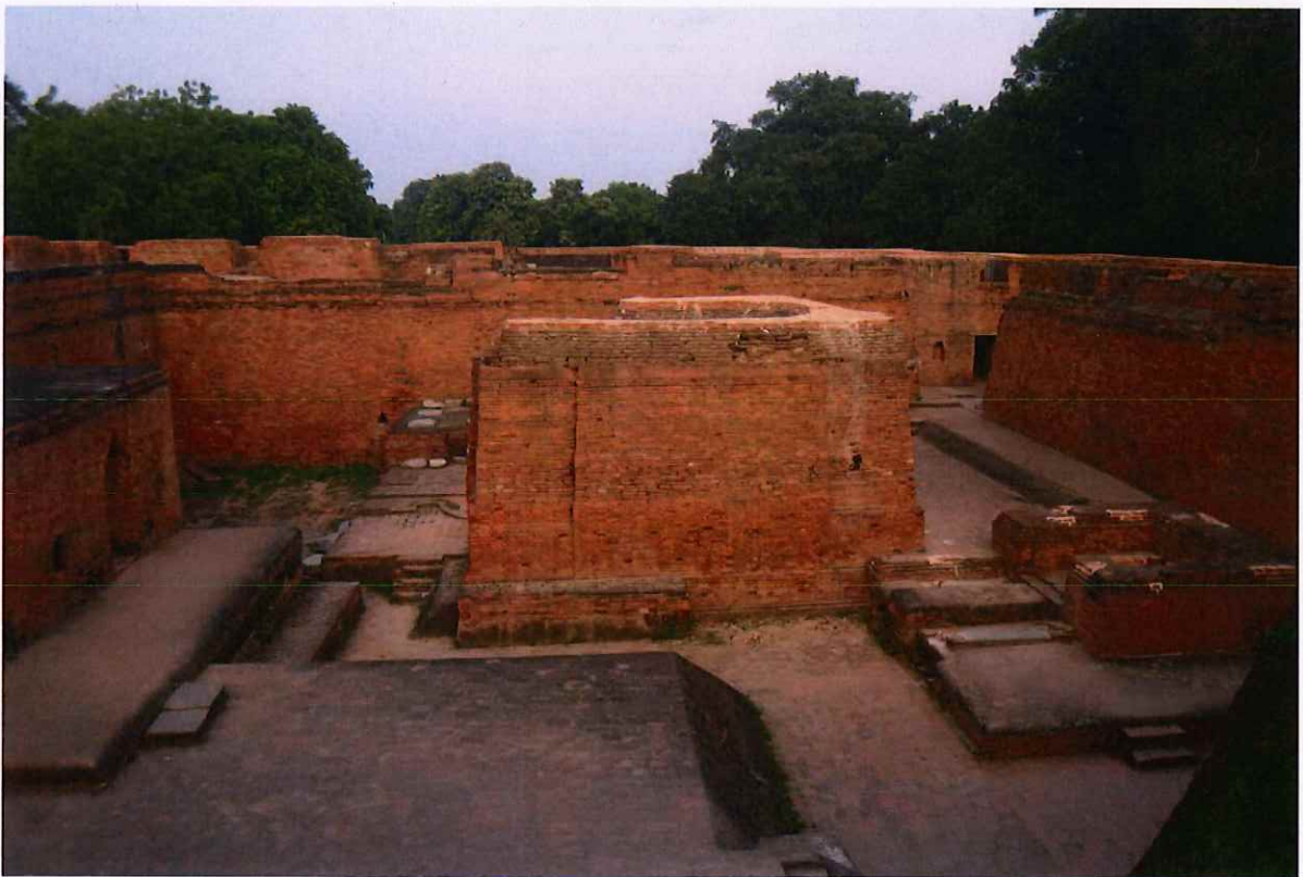
Structural Conservation at Monastery 1 (after)
