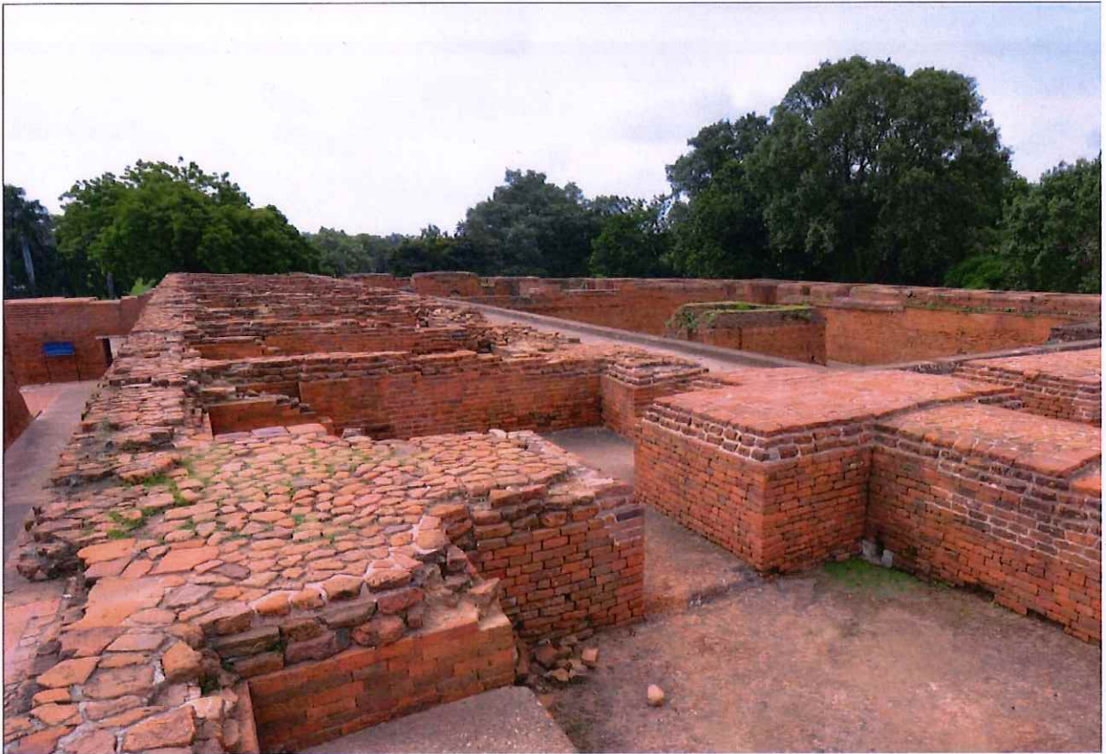
Structural Conservation at Monastery 1 (before)
