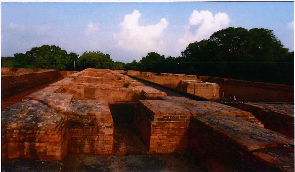
Structural Conservation at Monastery 1 (after)
