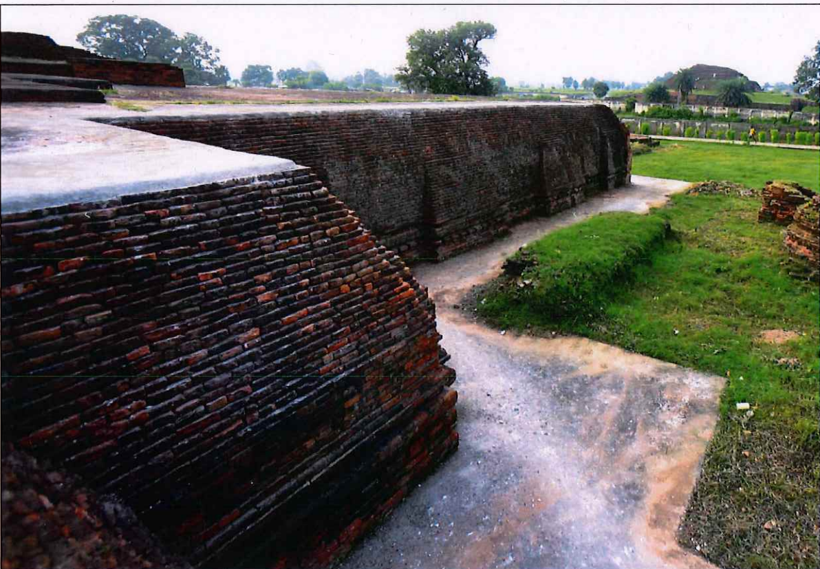
Structural Conservation at Temple site 13 (after)
