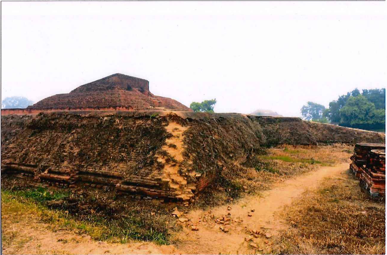
Structural Conservation at Temple site 13 (before)
