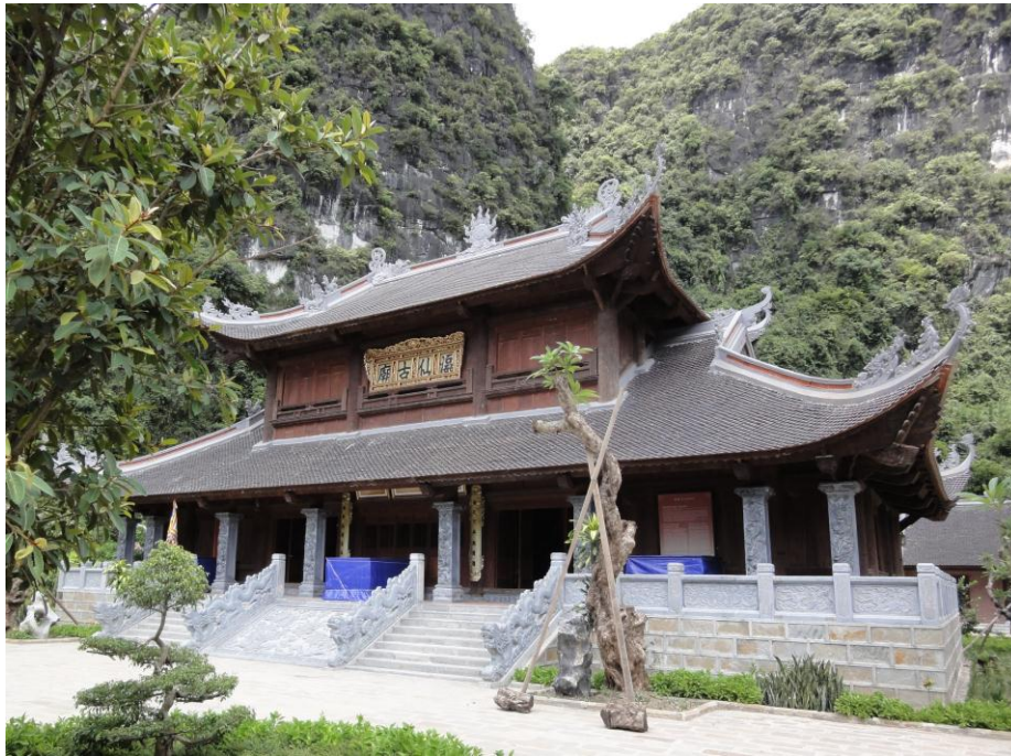
Figure 7: Vu Lam Royal ‘Step-Over’ Temple renovation and expansion (photo: P. Dingwall).
