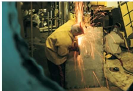
Fig. 2. Nuclear decommissioning worker wearing air-fed plastic suit underneath heavy leather overcoat, and multiple layers of gloves, while using power tools to cut legacy nuclear plant contaminated by alpha-radiation emitting substances, such as plutonium dust. The leather coat protects the plastic suit from being punctured by hot sparks during cutting. Maximum 2hrs work per day is possible, due to extreme discomfort and heat exhaustion as the suit fogs and fills with sweat. Image courtesy of Sellafield Ltd.
