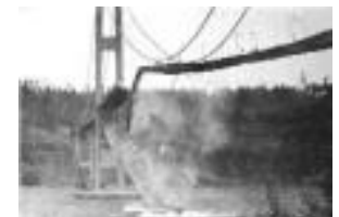
Tacoma Narrows Bridge shaking itself apart because it was too springy and started to resonate in the wind
