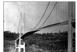
Tacoma Narrows Bridge in the wind
