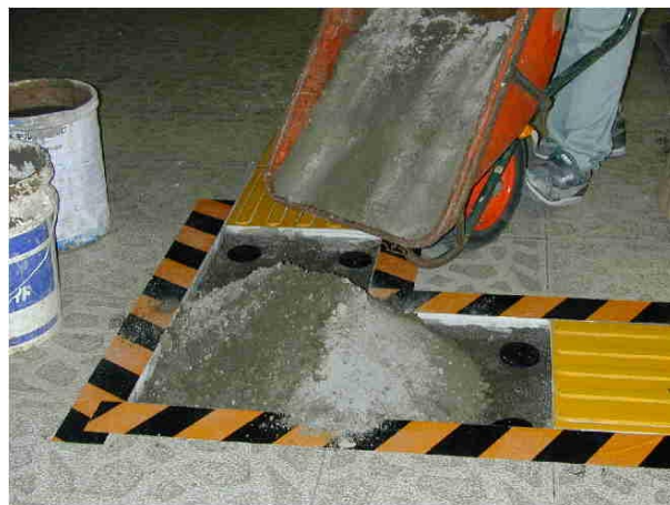
Figure 8: RF-ID tags embedded under the guide tiles on the station floor
